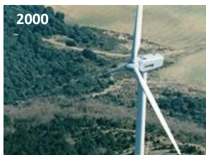
2000 - 1,300 kW wind turbine prototype
